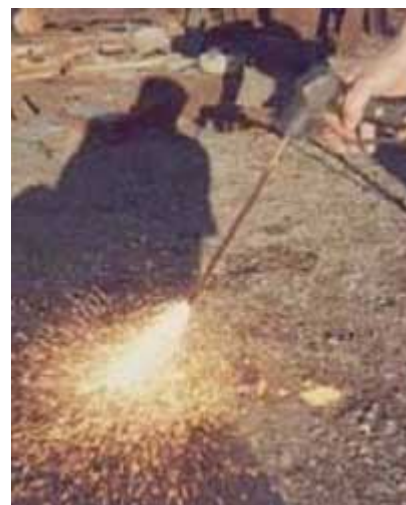
4. Within 5 seconds cutting rod ignition is achieved.
